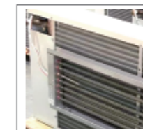
External re-heat coil
